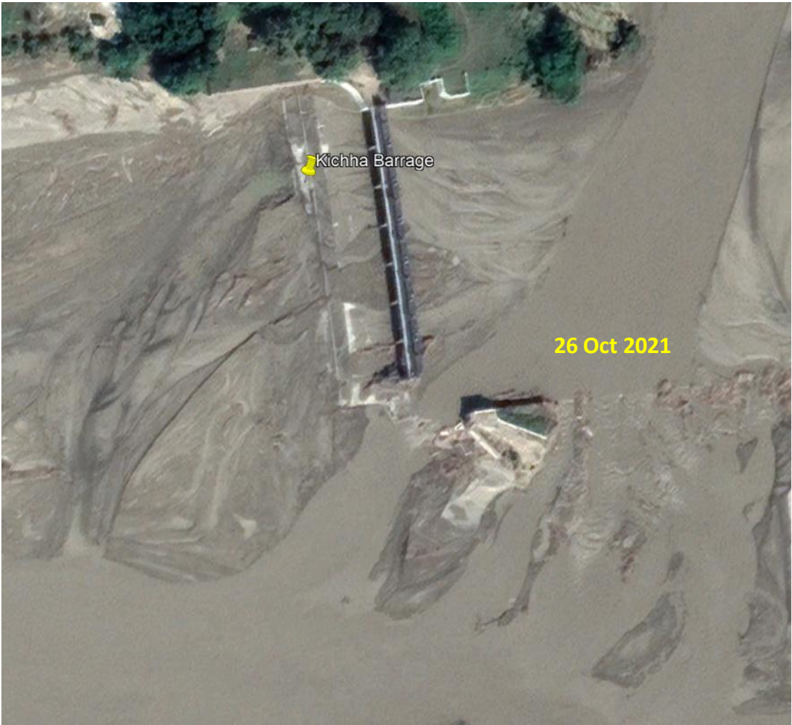
Figure 2.5: Satellite image showing damaged Kichha barrage as on 26 October 2021.
